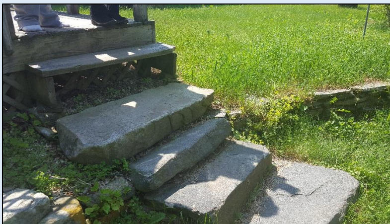
Photo 3 (top): The gap under Andrea's back door Photo 4 (bottom): The porch steps where Andrea's sons fell
